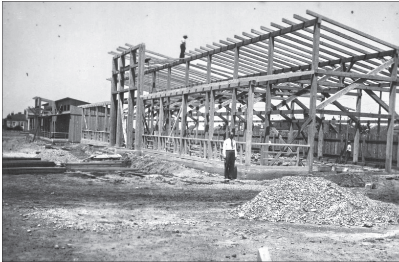
Figure 9. Construction of the pavilion (collection of Miloš Jurišić)
